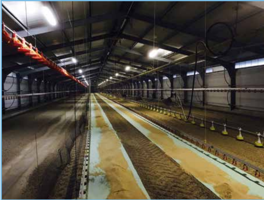
Installation tubes fluo compact
